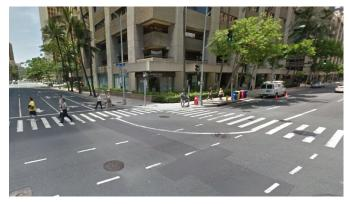
Figure 6.5: Lane extension striping guides left-turn King Street vehicles into the second-from-the-left lane on Alakea Street, which alleviates interruption from frequent Tow-Away Zone violations in the far left lane on Alakea Street.
