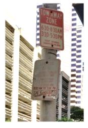
Figure 7.1: Faded Signs along Alakea Street which are difficult to read.
