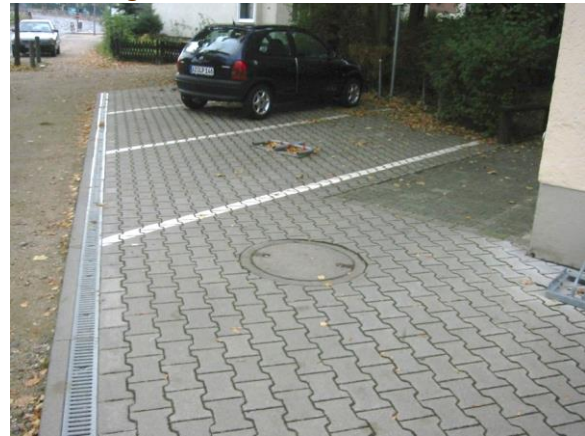
Figure 9-19: Permeable Paving and a Trench Drain in a Parking Area
