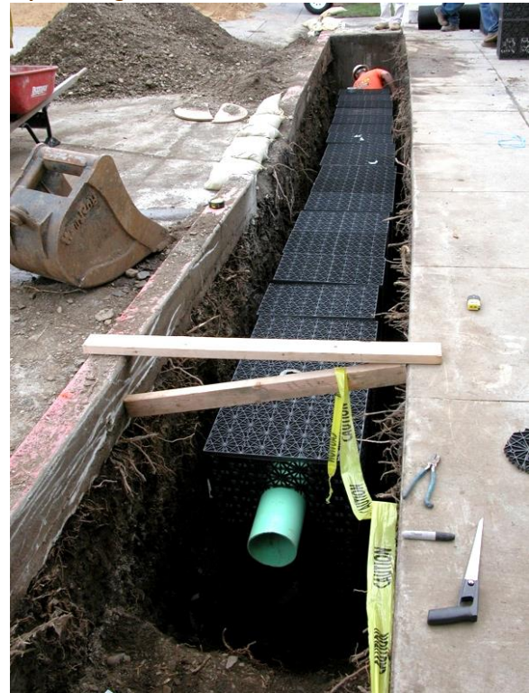
Figure 9-15: Infiltration Trench With Perforated Pipe During Installation
