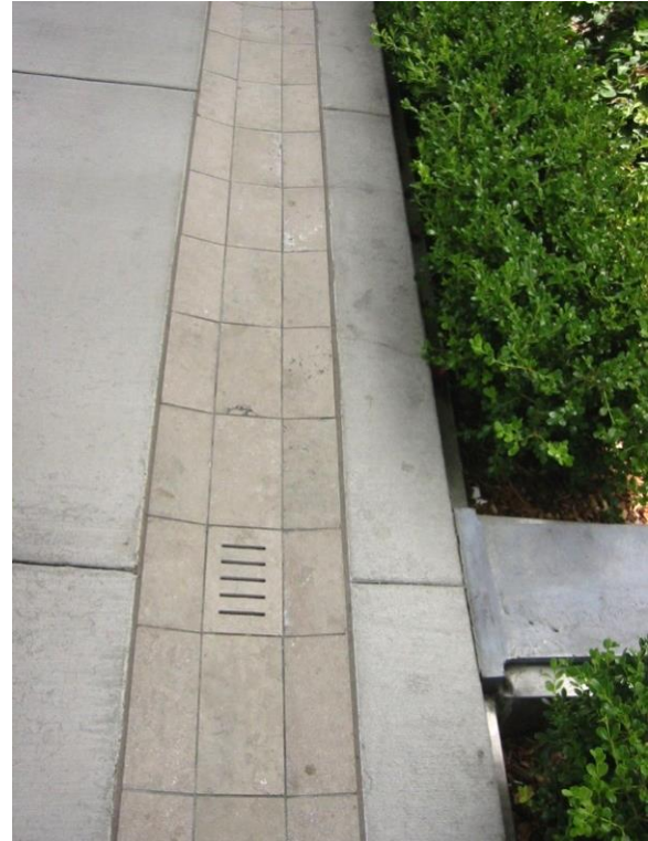
Figure 9-21: Constructed Swale With Drain
