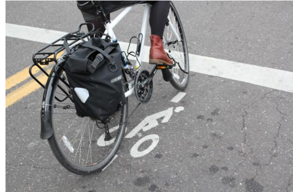
Figure 6-39: Bicycle Signal Detection Marking
