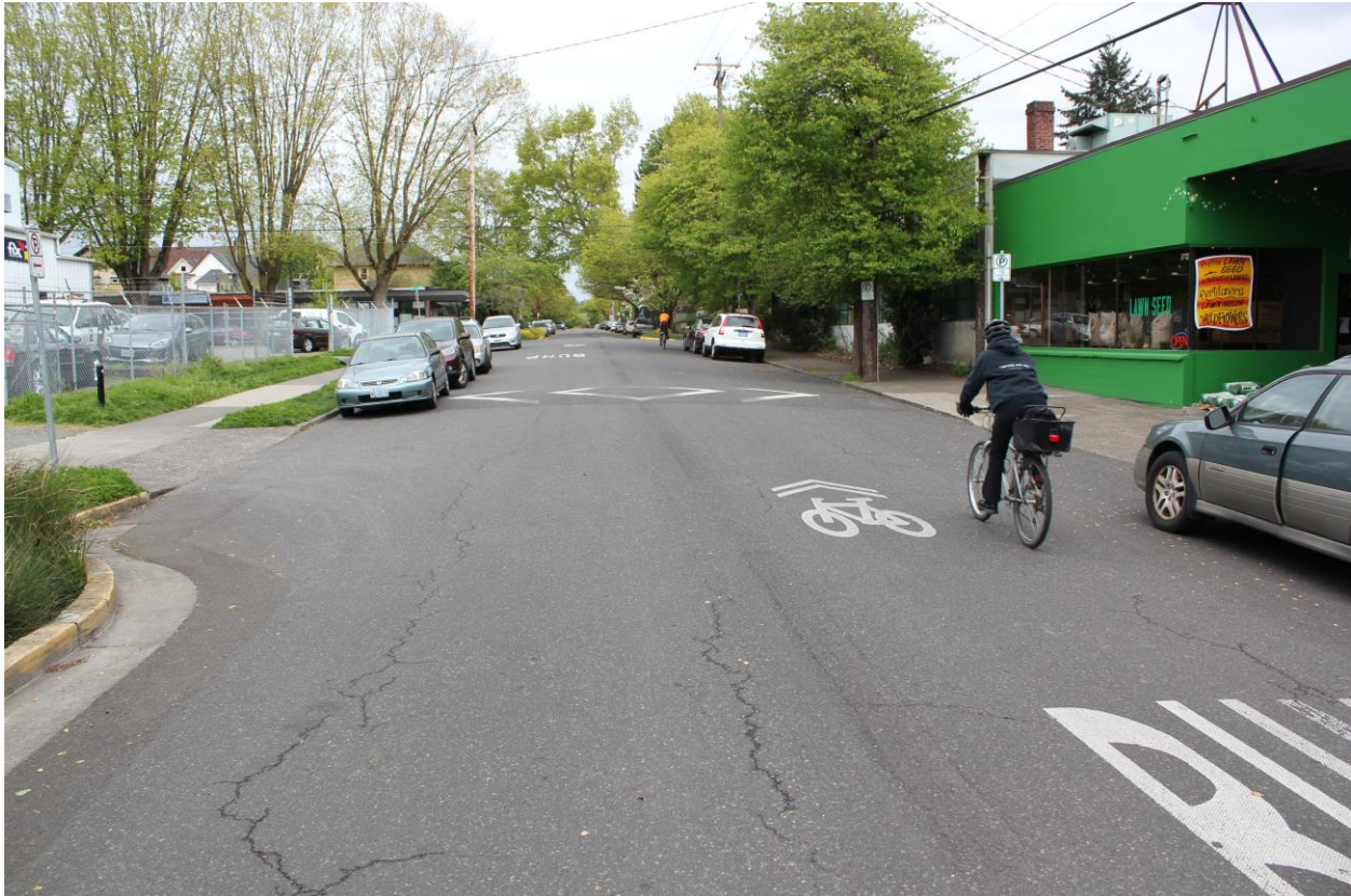
Figure 6-16: Traffic Humps, Bump Outs and Sharrows Along Bike Boulevard
