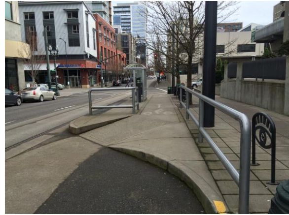
Figure 6-22: Bus Stop Islands Can Maintain Separation From Bike Lanes
