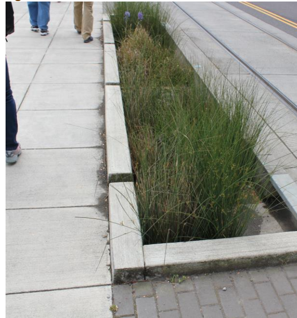
Figure 9-10: Sidewalk Swale with Curb Inlets
