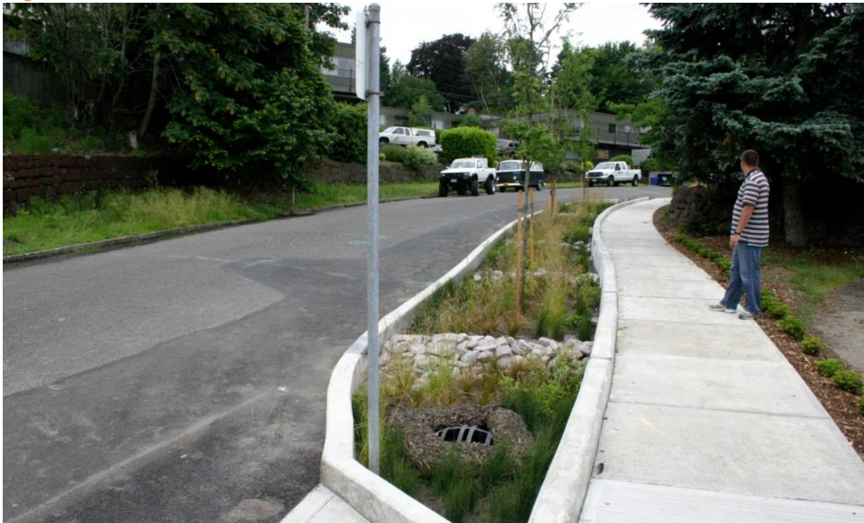
Figure 3-39: Mid-Block Curb Extension with Bioswale
