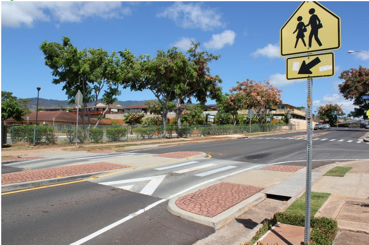
Figure 5-15: Raised Crosswalk With Median and Bulb Out
