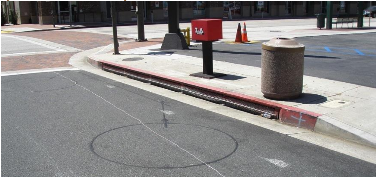
Figure 9-23: Curb Inlet Grade Catching Debris
