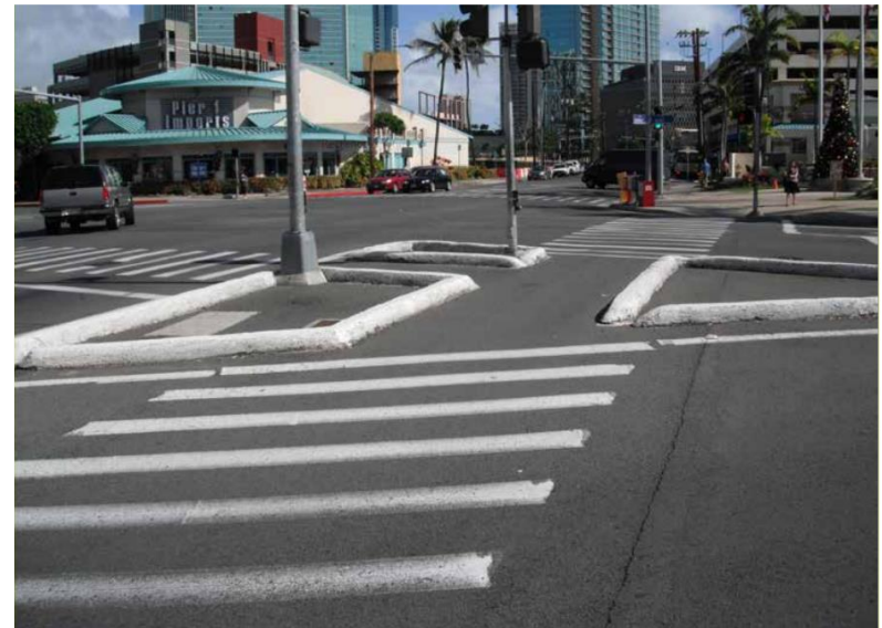
The median refuge island provides a cut-through for accessibility and shortens the crossing distance at this wide intersection in Honolulu.
